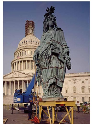
*The bronze statue was removed by helicopter to the East Front plaza for restoration in 1993. Surface corrosion and discoloration of caulk in the seams were the most visible signs of its exposure to the elements for over a century.*
